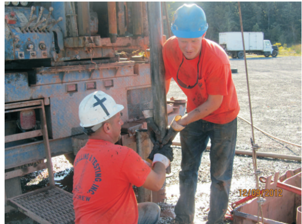
Aquifer Drilling and Testing Inc. extracting core after removal of drill bit.
