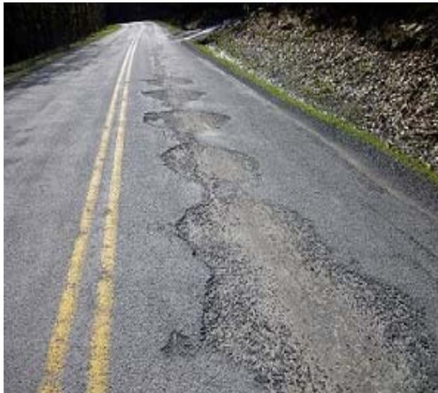
As the roads are being swept simultaneously they are being assessed. Asphalt road surfaces have oxidized to the point of little or no stone retention, combined with the harsh weather conditions of this past winter freeze/thaw resulting in wearing surface unraveling of over 27 miles to date. (More to follow). Ex: to include but not limited to: Chadderdon Road, Edison Timmerman, Joel Austin, M. Simons, Frank Hitchcock, etc.
