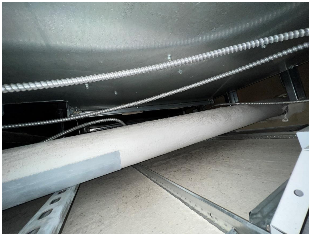
Photo 4.0 VSMG on fiberglass pipe insulation above the suspended ceiling in the Kitchenette area.
